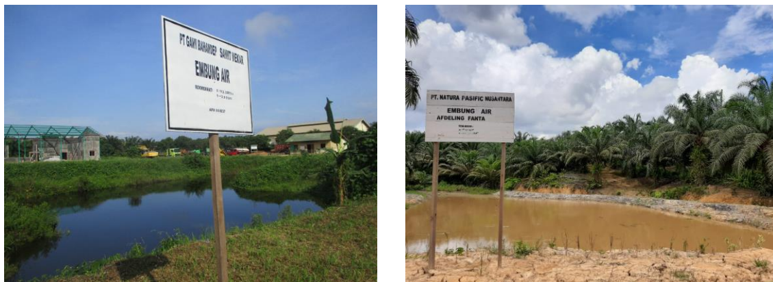
Figure 55. TAPG’s water dam
