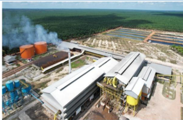
Figure 17: NSSS' first mill (NSP) – 60 tonnes per hour
