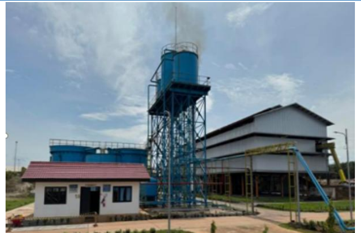
Figure 18: NSSS' second mill (BSP) – 60 tonnes per hour
