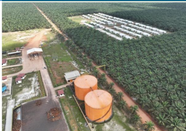
Figure 20: BSP's direct piping system
